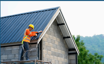
Maintenance Building Naming Rights
